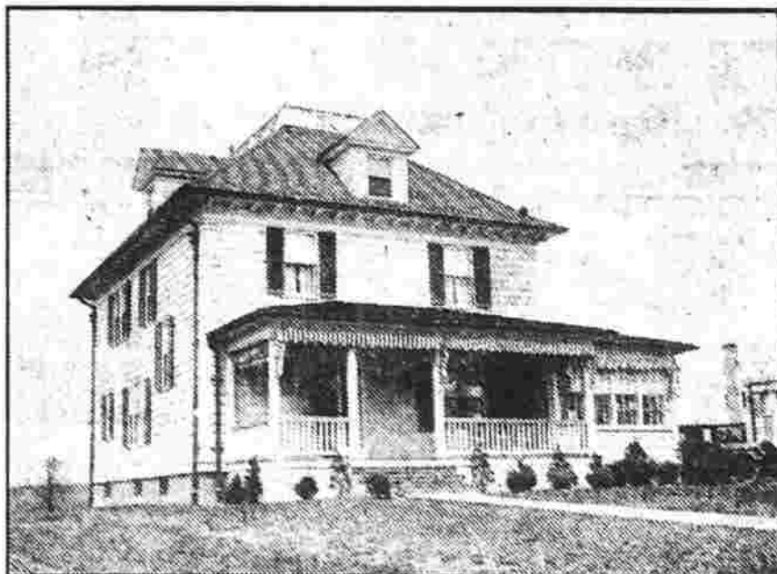
Residence of Charles E. House, East Center Street
